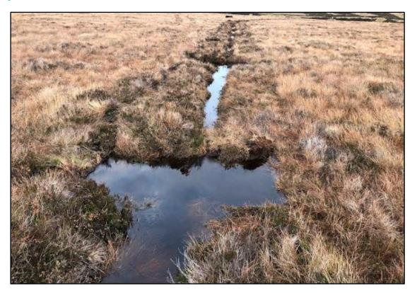
Plate 2-2. Example of peat dams to be used for on-site drain blocking. This will re-establish and maintain a hydrological regime for the required peatland rehabilitation.
